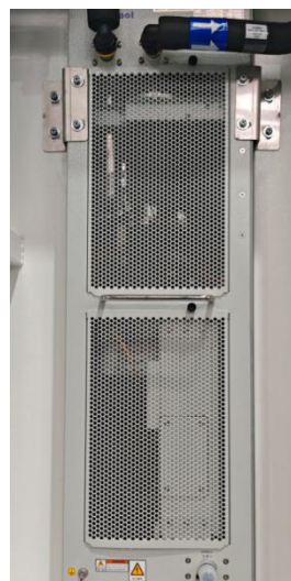
Figure 7-3 Liquid-cooled Chiller Unit Filter
